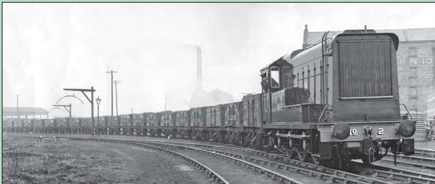
Above: One of the 'classic' diesel shunting locomotive pictures of all time, Great Western Railway No. 2 at work. The image was recorded when the loco was brand new in the mid-1930s, during a demonstration of 'modern' diesel shunting power. This image clearly shows that no train brake equipment was fitted and that the bodyside ladder was installed on this side of the loco only, and not as shown in the drawings. CJM-C
