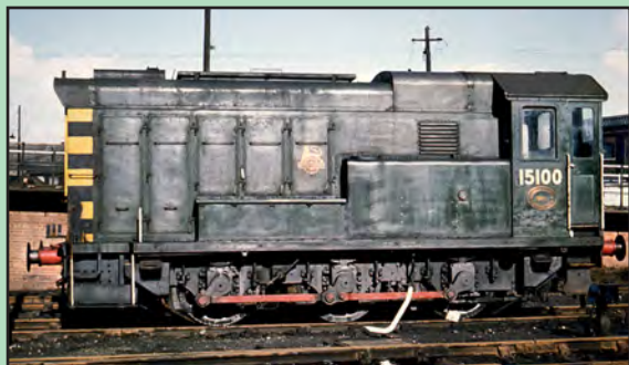
Below: In summer 1963 No. 15100 visited Derby when this illustration was taken. Note the large cast oval worksplate on the cabside. www.colour-rail.com / A. E. Doyle
